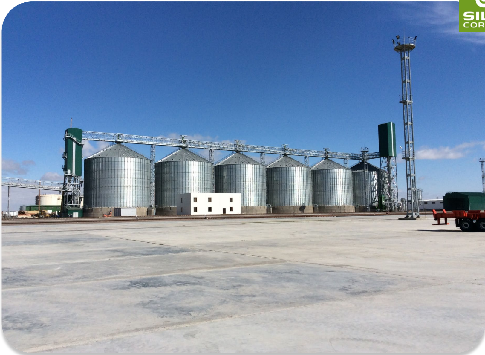
2015 AKT - KAZAKHSTAN: 6 silos mod. 27,50/18 - Total capacity: 62.000 T
