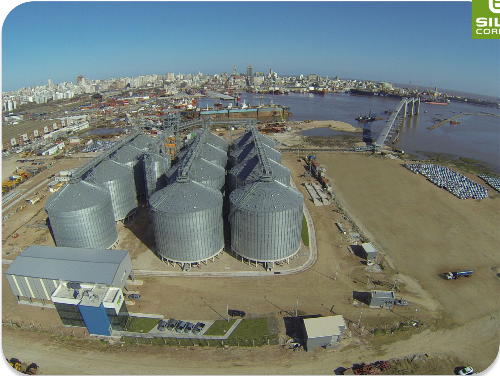
2015 OBRINEL - URUGUAY: 12 silos mod. 27,50/17 - Total capacity: 121.000 T
