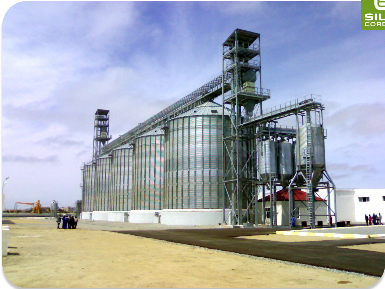
2007 BAKU – AZERBAIJAN: 5 silos mod. 16,81/14 – Total capacity: 15.000 T
