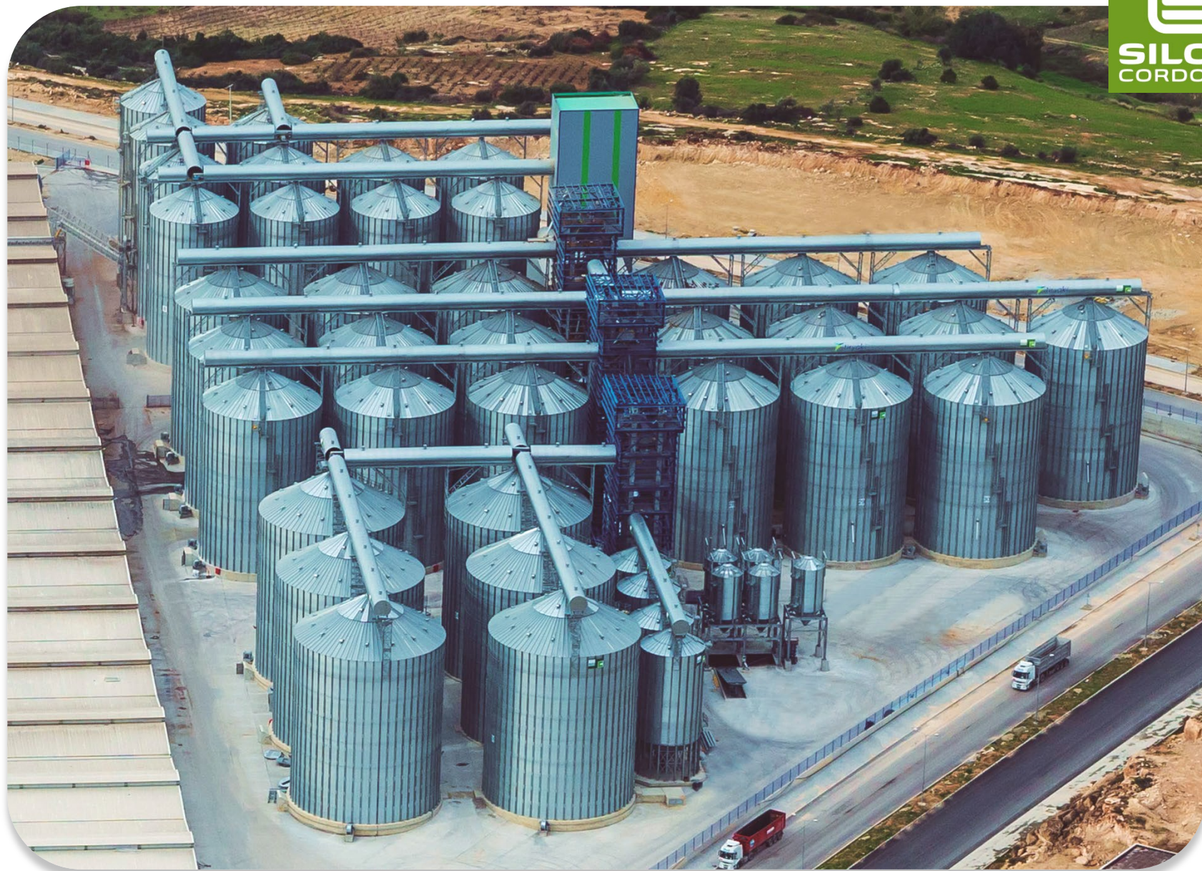
2013 TIRYAKI - TURKEY: 19 silos mod. 18,33/22 – 11 silos mod. 14,51/22 – 27 truck load silos mod. 4,65/6 – 6 silos mod. 21,39/22 – Total capacity: 200.000 T
