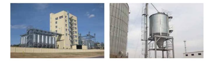
For agricultural facilities, feed mills or flour mills, the silos available range from 2.55 m in diameter to 4.65 m with capacities ranging from 12 m<sup>3</sup> to 116 m<sup>3</sup>. For industrial facilities with silos for truck or rail dispatch, we recommend silos with a diameter of at least 4.58 m and capacities ranging from 80 m<sup>3</sup> to 400 m<sup>3</sup>, upon request.
