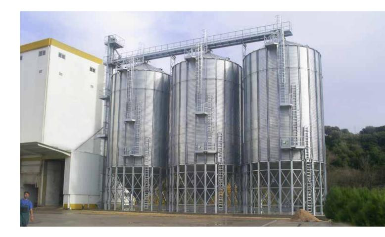
They are designed to store grains, seeds, legumes, pellets and other products that require special storage conditions. The stored product stays off the ground to prevent moisture gaining and lower the possibility of breakage.
