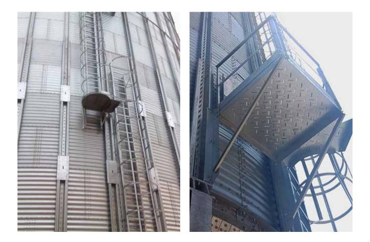
All of the means of access and maintenance on our silos have been designed for user safety and ergonomics and are designed pursuant to **standard UNE-EN ISO 14122-2.**
