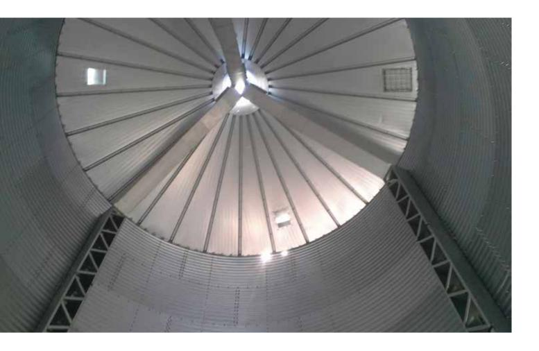
**Internal sledge** is an inner conduit situated on roof and wall of the silo to make the product slide down homogeneously to prevent breakage during loading (of the silo).
