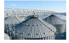
**Rest platform** on silo hatch is an optional element and fosters the connection supervision work between the machinery and the silo.
