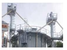
The **perimeter handrail** is a structure that enhances safety when doing maintenance work on the silo roof.
