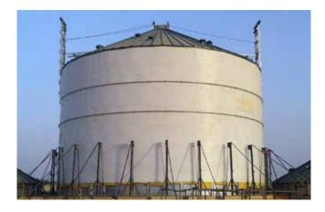
Double sheet insulation: For roofs, wall rings or the cone. The outer sheet can be pre-lacquered, preferably in white.
