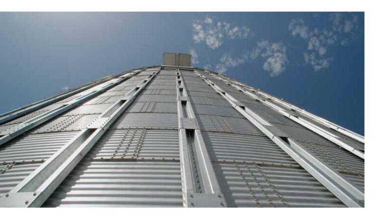
We use steel with a **yield strength ranging** from 450 MPa for wall rings and for stiffeners. Silos Córdoba is the first silo manufacturer to use Z-600 galvanised steel as its manufacturing standard. This coating contains 600 gr/m<sup>2</sup> of Zinc and is equivalent to a thickness of 42 micras per side which makes it longer-lasting even in the most aggressive of atmospheres (as established in Standard ISO 9223).
