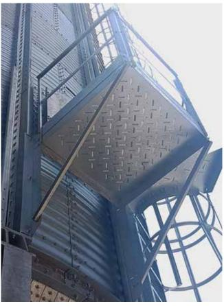
All of the means of access and maintenance on our silos have been designed for user safety and ergonomics and are designed pursuant to standard UNE-EN ISO 14122-2.
