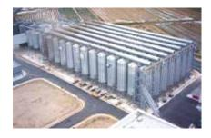
This type of silo not only brings economic savings, as no sweeping machine is necessary, but also simplifies the foundation work which considerably reduces the building costs and streamlines assembly work.
