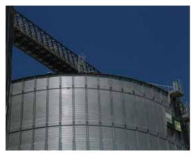
Wind-Ring allows silo to maintain its cylindrical shape without any effect from wind loads which offers rigidity and safety. They may be installed on the roof or on the wall ring depending on the diameter and height of the silo.
