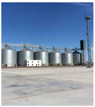
Our silos with a cylindrical body and 30° sloped roof are designed to store grains, seeds and pelletized products. Silos Córdoba engineering team designs its silos pursuant to various standards in order to adapt to its customers' needs including European EUROCODE and US ANSI standards.
