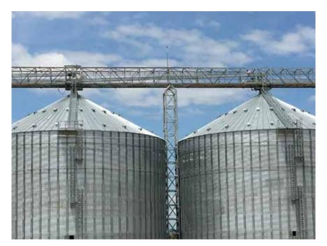
Silos Córdoba **roof vents** guarantee proper silo ventilation and the meticulous design prevents the entrance of water even in the most adverse of conditions. They may also be supplied with an anti-snow kit.
