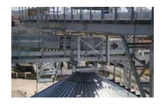
Cap support supports the catwalk and is placed above the top cover of the silo roof. There are different types based on the machinery performance and type of catwalk.
