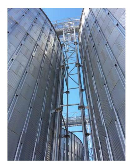
**Elevator towers** are modular bolted and welded structures made with double-T laminated profiles in galvanised steel. They offer stability, easy access to the catwalks and make for safer elevator maintenance. With a floor that can be walked on, electro-welded grating and maintenance platforms including securing tensioners.
