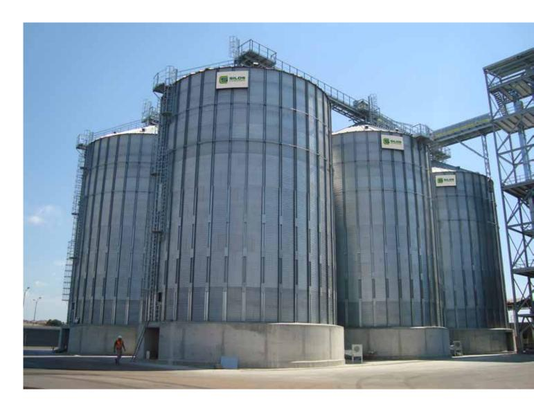
Our silos, either flat or hopper bottom, are used for extended storage of large quantities of grain, seeds and granulate products
