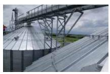
The **lateral support** is bolted to the silo stiffeners. Used for light machinery in silos of up to 24 m in diameter. Additionally, an oblique support can be added to the lateral support depending on the silo and catwalk model.
