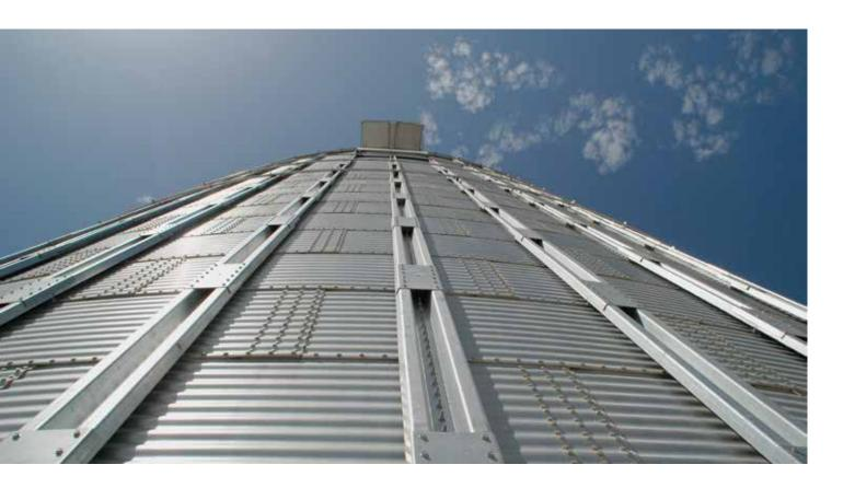
We use steel with a **yield strength ranging** from 350 MPa for wall rings up to 600 MPa for stiffeners. Silos Córdoba is the first silo manufacturer to use Z-600 galvanised steel as its manufacturing standard. This coating contains 600 gr/m² of Zinc and is equivalent to a thickness of 42 micras per side which makes it longer-lasting even in the most aggressive of atmospheres (as established in Standard ISO 9223).
